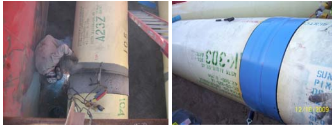
Joints being welded, heat-shrink sleeves
