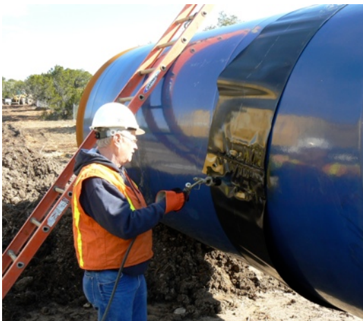
Infield Heat Shrink Sleeve Application
