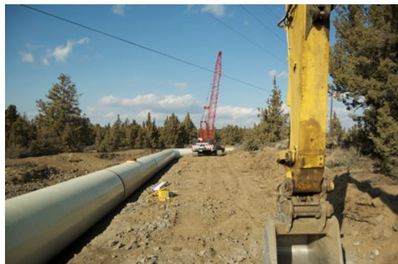
Pipe Laying Operation at Juniper Ridge
