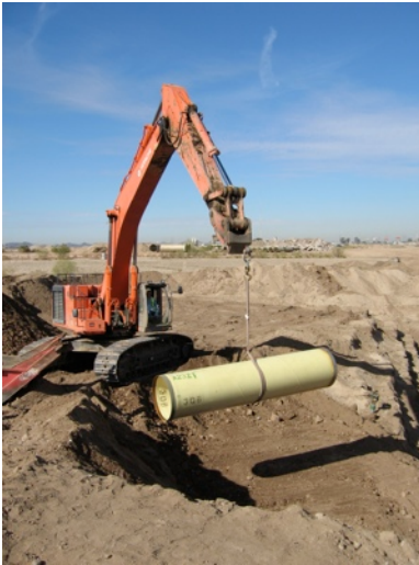
42" Welded Steel Pipe Installation
