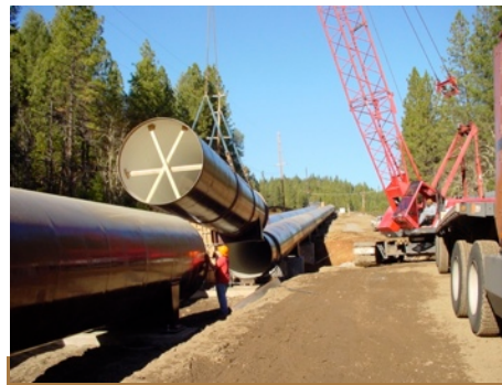
78" Welded Steel Pipe Installation
